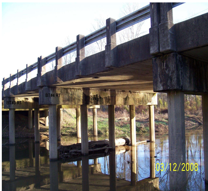
PHOTO 3 Description Bent 4 ahead, cap is cracked with 3' spall
