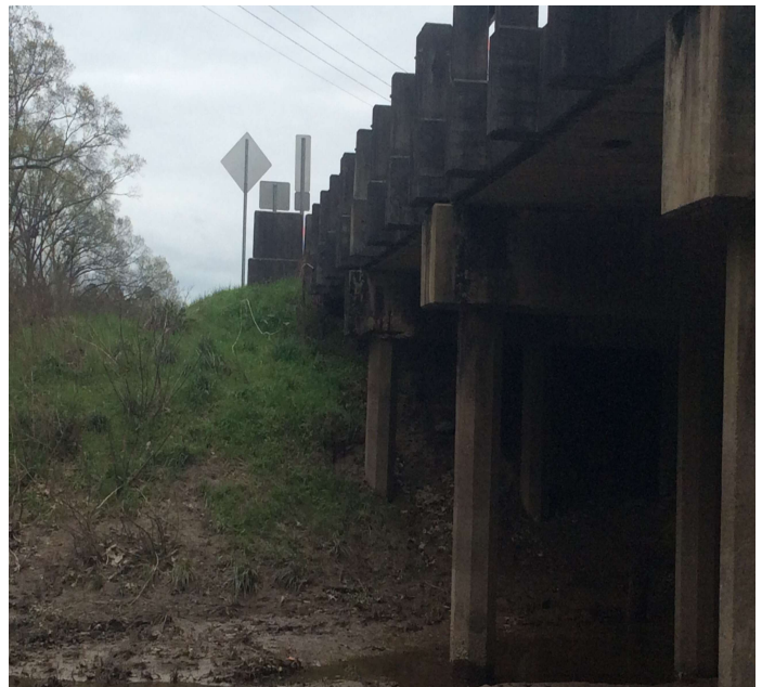
PHOTO 2 Description Bent 6 cap spalled
