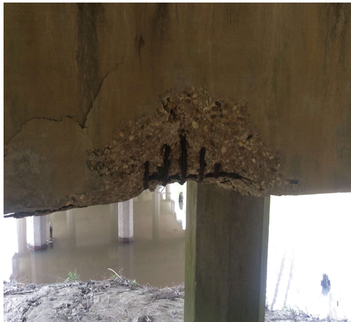
PHOTO 1 Description Bent 2 cap spalled with exposed steel.
